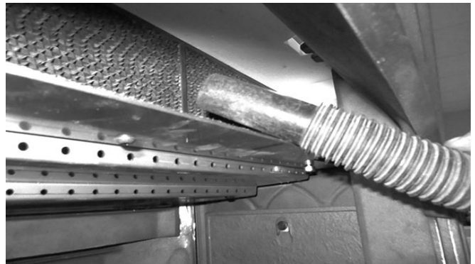
Fig. 18. Vacuum the combustor cells after brushing.
