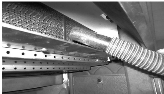
Fig. 18. Vacuum the combustor cells after brushing.
