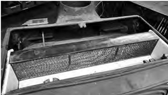
Fig. 24. Left and Right Side insulation panel removal and replacement.
