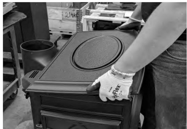
Fig. 21. Remove the top plate from stove.
