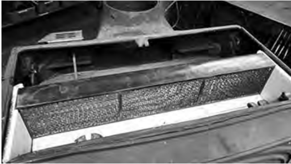
Fig. 23. Lift combustor from the chamber.
