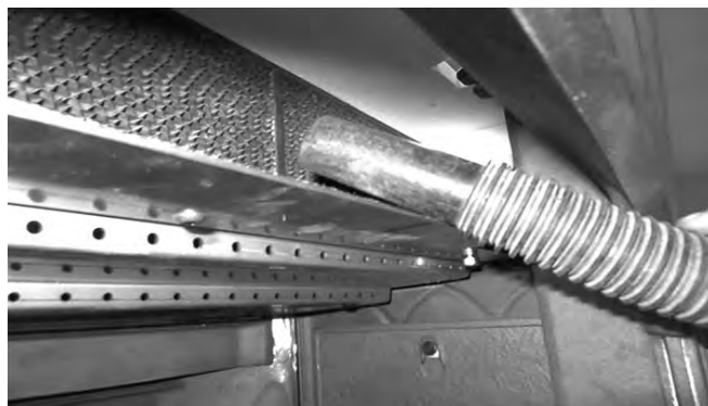
Fig. 18. Vacuum the combustor cells after brushing.
